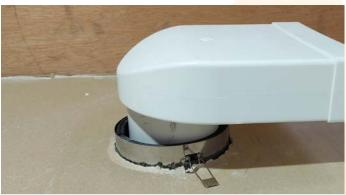
3. From the underside push the Quelfire CFC up into the aperture around the PVC duct ensuring the spring clip clamps fully back onto the plasterboard and that the Quelfire CFC is clamped tight in position.
