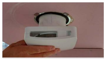
5. Connect the ceiling fan to the vent duct
