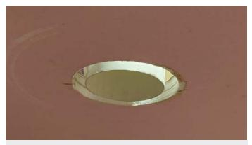
2. Centralise the PVC duct spigot within the hole.
