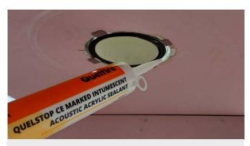
4. Make sure the gap between the CFC and the plasterboard is clean of any debris and remove dust from all edges. Seal the small gap between the CFC and the plasterboard, and around the power cable with QuelStop Acrylic Sealant.
