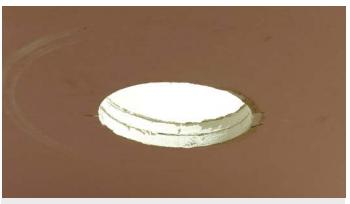
1. Cut the plasterboard aperture to suit the PVC duct spigot as per the table above.
