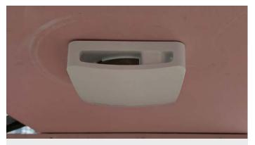
6. Install the ceiling fan to the plasterboard with correct screw fixings in accordance with the ceiling fan manufacturers requirements.
